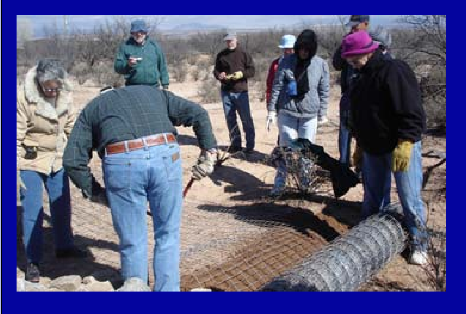
Dave Matthews, NRCS , gives tips on using 12 gauge, hinged-joint wire to build structures.
